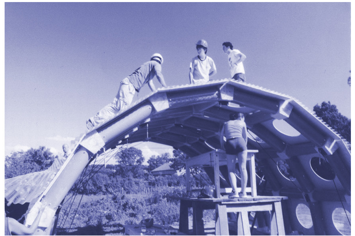
Figure 5 Earth Dome in Hill-Holt Wood covered in car tires and a vault by Shigeru Ban supported by paper tubes. Both projects were possible because of low-tech's distinctive feature which is encouragement of self-built and experimentation with cheap non-standard materials.
