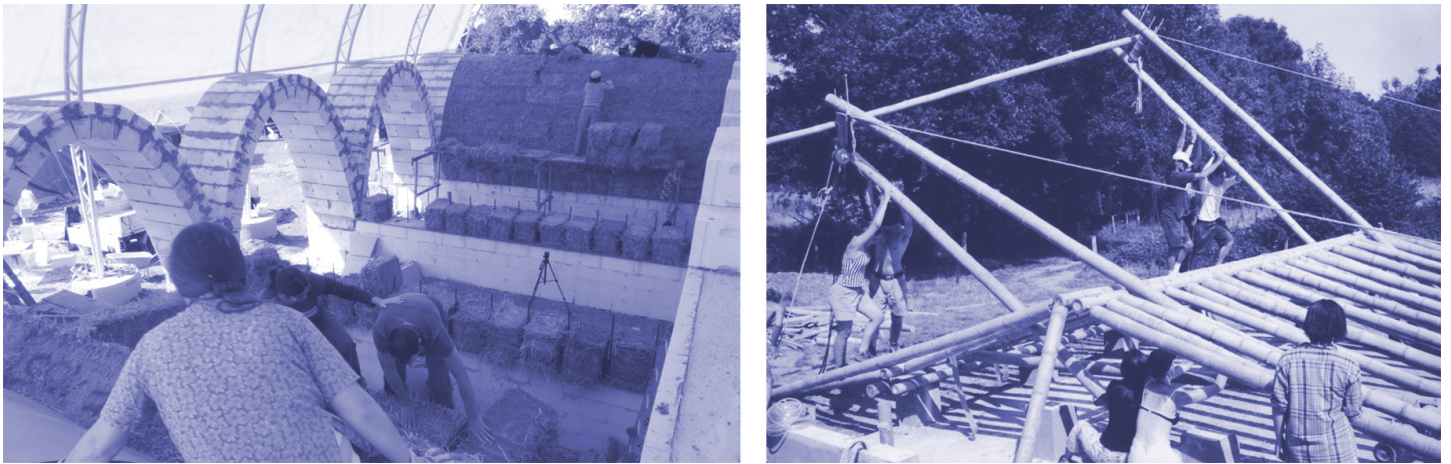
Figure 6. Straw vaults in Wangelin (by Gernot Minke) and Bamboo House in Boisbuchet (by Simon Velez). Those projects, like many other low-tech projects, were possible because volunteers are attracted to natural building sites.
