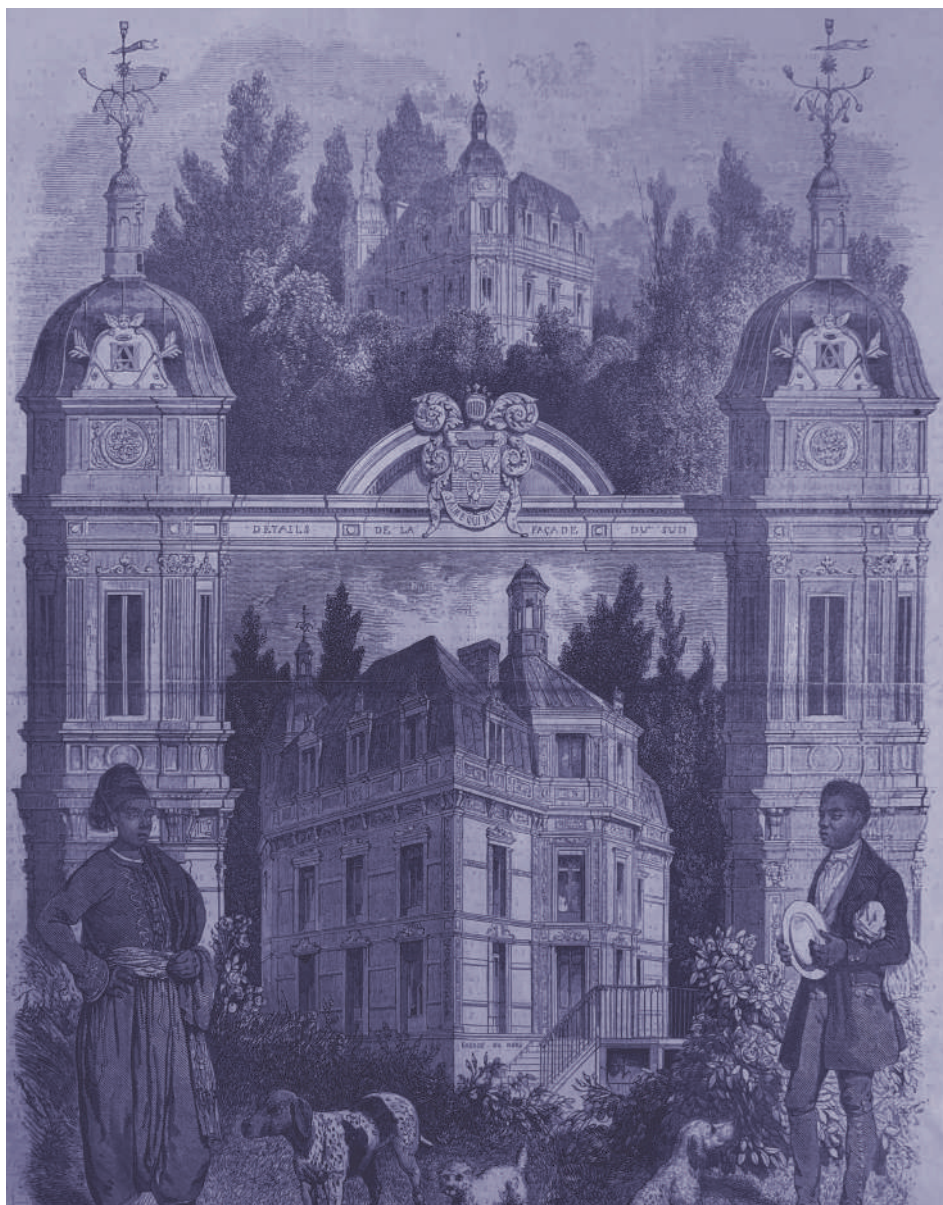
Fig. 2 – Monte Cristo north façade and details of south façade.
