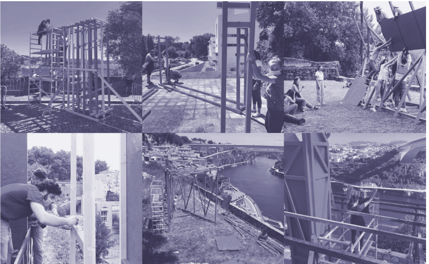
Fig. 9 - Work in progress construction weeks of all teams. Follies 1 to 6, from top left to bottom right.
