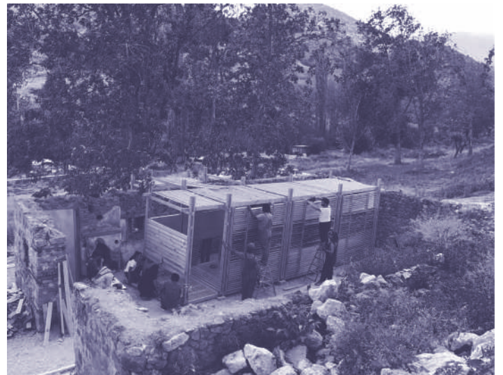
Fig. 3 - Construction of the folie, Merzifon, 2017
