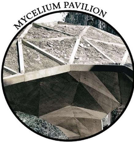
Ephemeral pavilion made of mycelium pieces with parametric patterns that you can put together and then disassemble to take it away from that place so that it does not have a bad impact.
