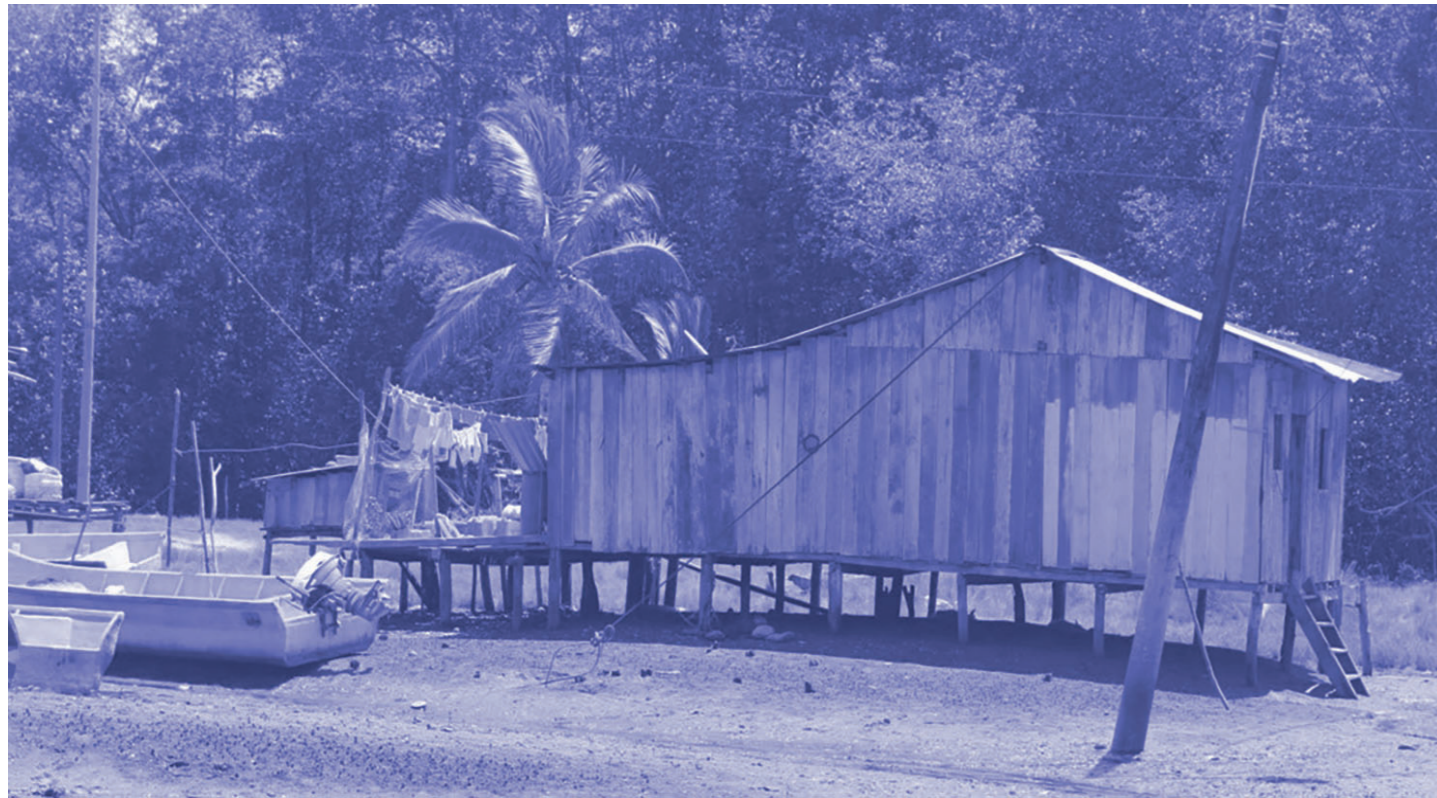
Fig.6 – Typical house. Author source.
