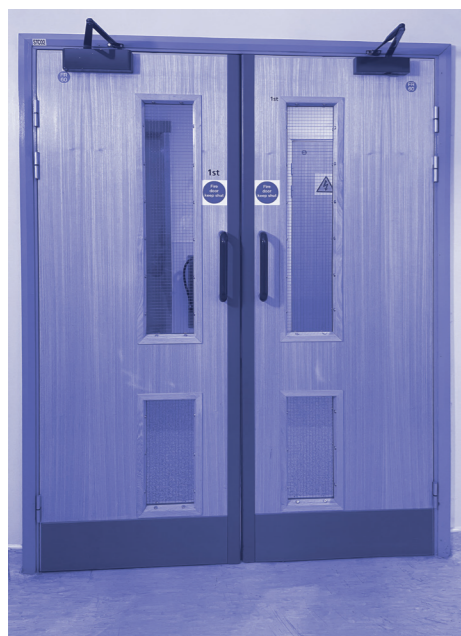
Fig.7 - Contrast in doors, trim, walls and floor.
