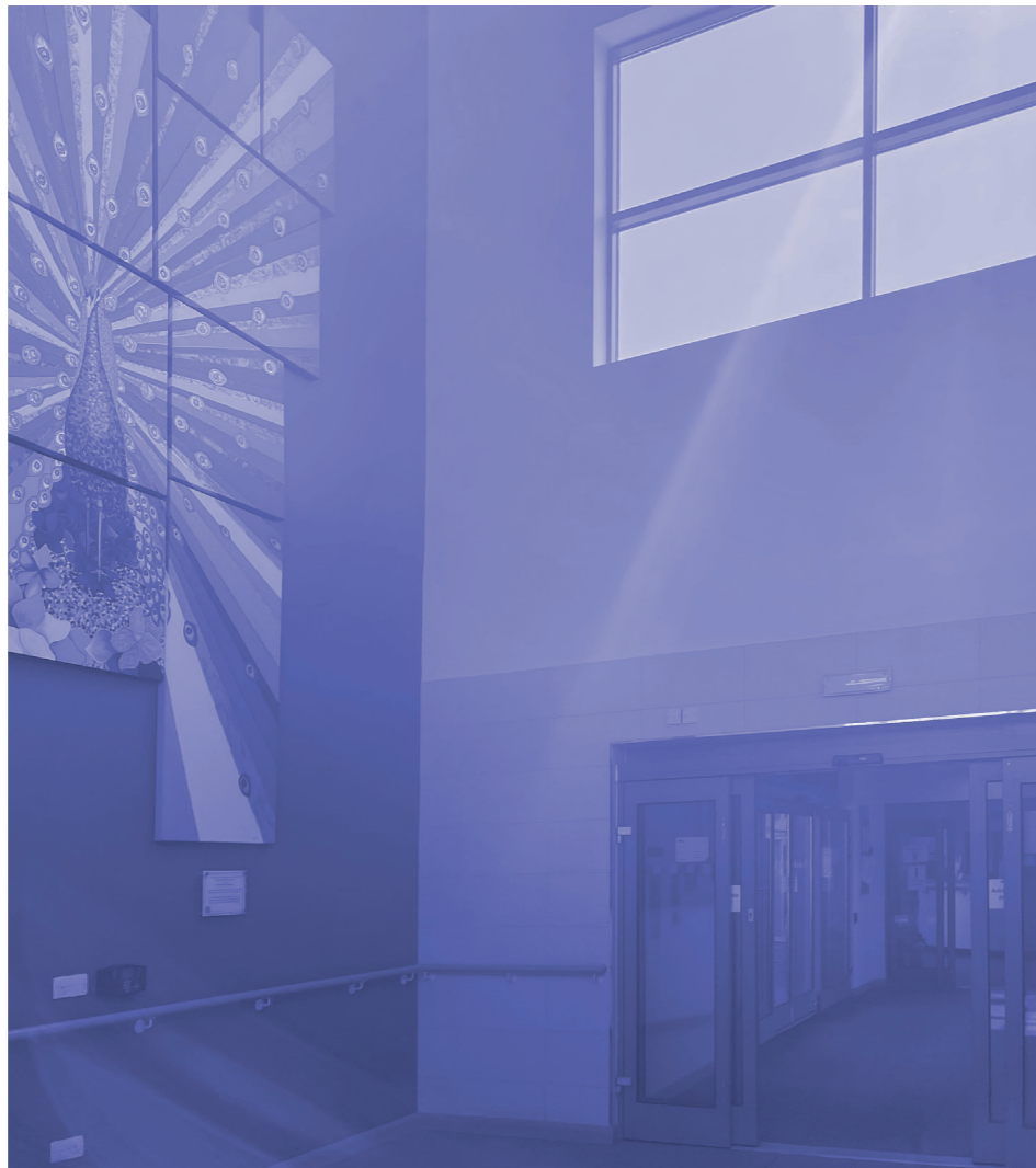
Fig.6 - Natural lighting coming in from above to provide a diffuse light.
