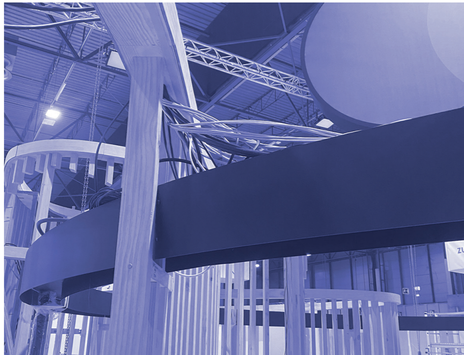
Fig. 9 - The black central ring as wiring distributor.
