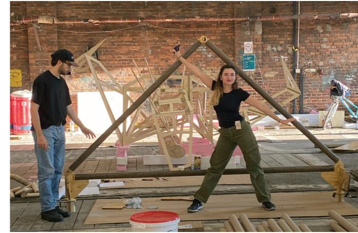
1. Production of the Eco House Pavilion.
