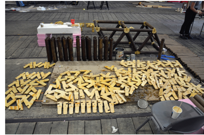
1. Timbre joints and paper tube truss of the Green Gaya Pavilion.
