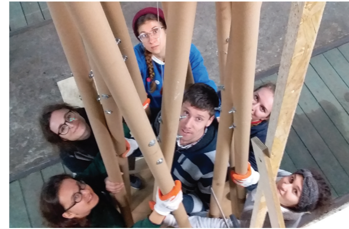
1. Assembly process of the tower.
