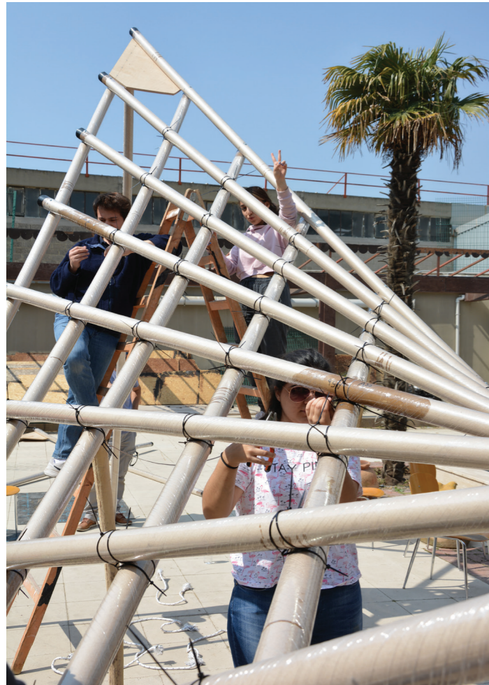
1. Assembly process of the structure.
