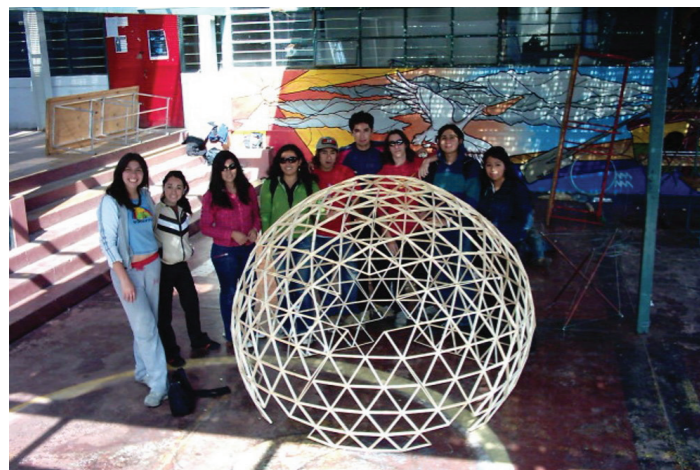
3. Timber prototype of Fuller's Geodesic Dome.
