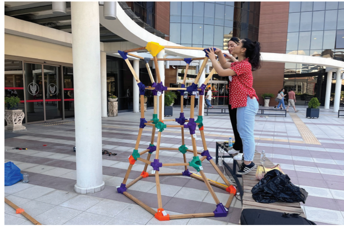
1. Assembly process of the column section.
