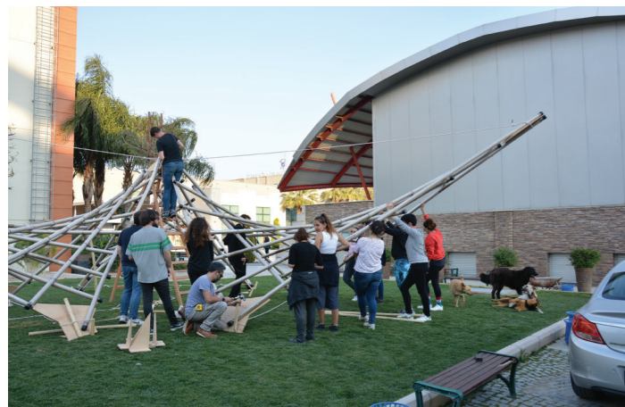
2. Installation of the hy-par structure in the university campus.
