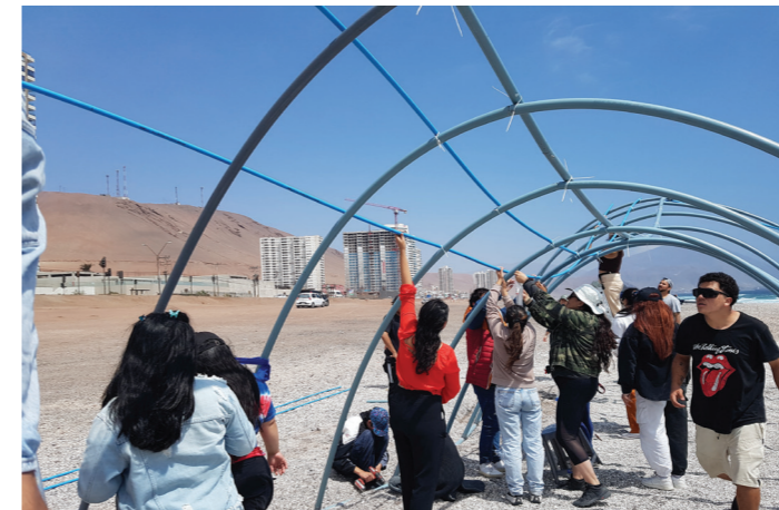
2. Assembly process of the Wind Machine II.
