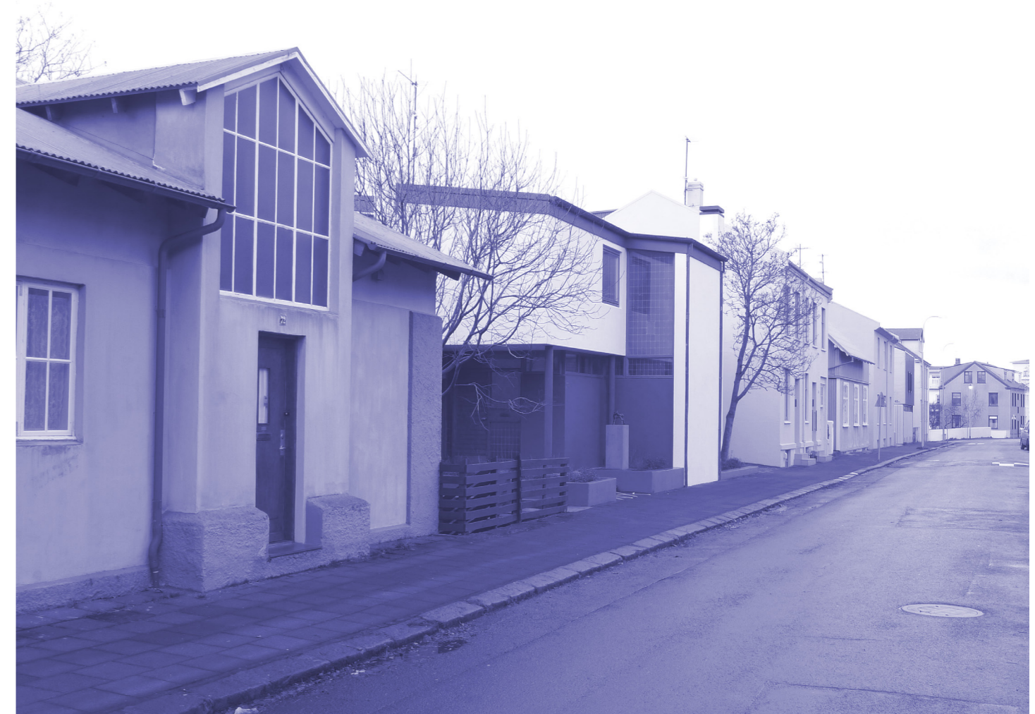
Fig.8 - The house is singular for its respect for the preexisting environment in grown street, receding from the street and creating a sheltering entrance from the wind and rain (© The Cultural Heritage Agency of Iceland)
