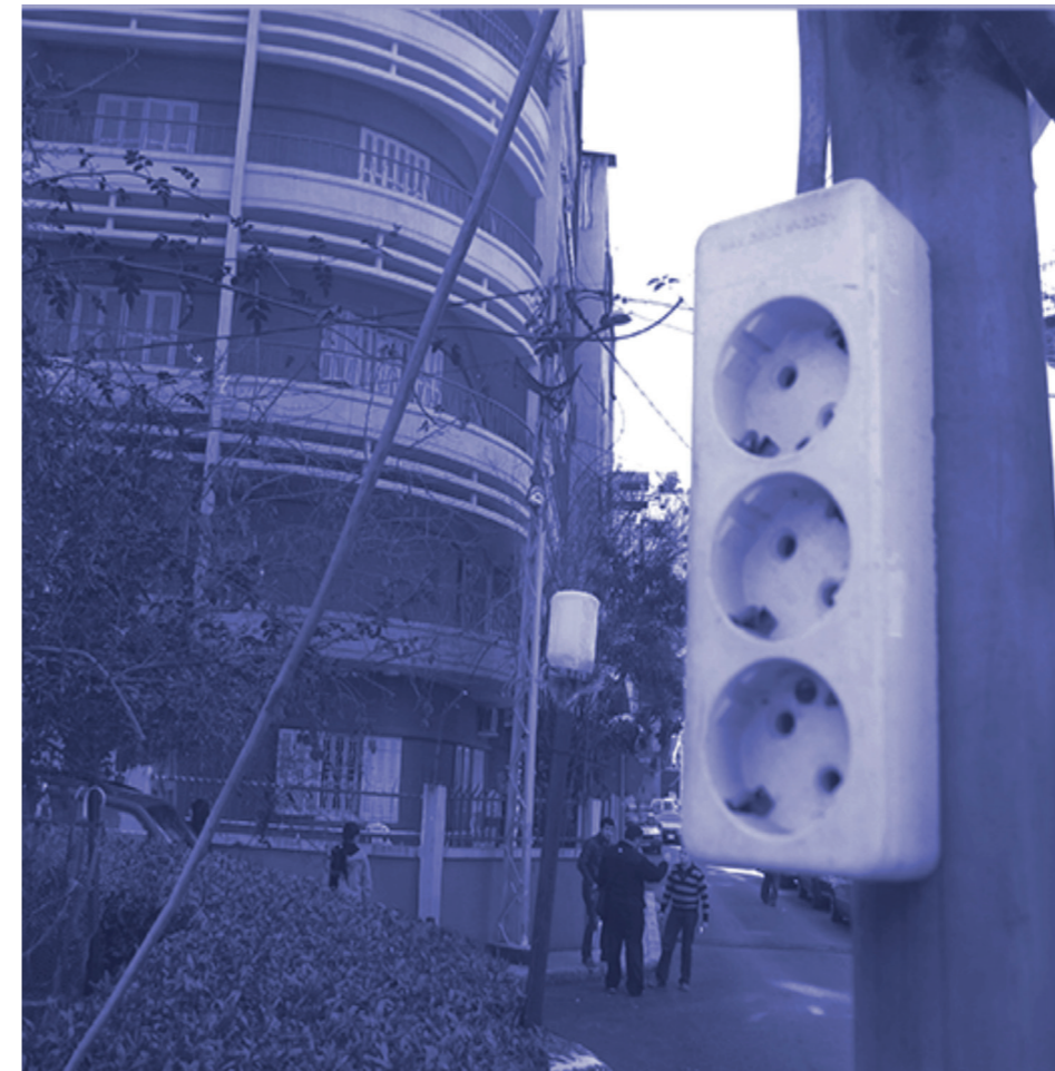
Fig.9 - Lighting pole and electricity socket (2012).
