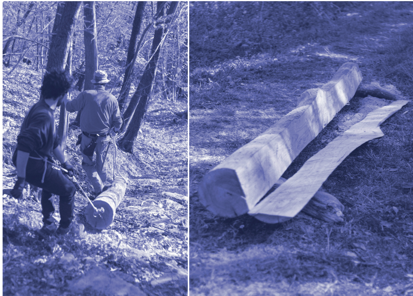
Fig.3 and 4 - Collecting logs in the forest as part of the construction process. The dead standing trees were felled and sectioned into movable lengths, then guided downhill out of the forest. As this primitive method of transportation tends to leave surface marks due to ground friction, the final processing of timber was made on site. 2025. Photos by the author.
