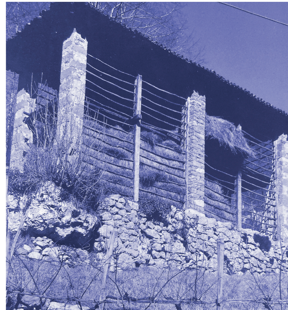
Fig.7 - Example of a Kozolec with stone pillars. (Rucli 1998).
