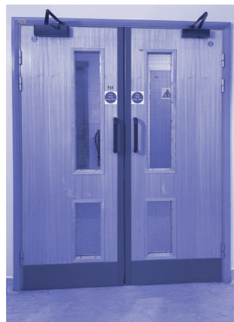
Fig.7 - Contrast in doors, trim, walls and floor.
