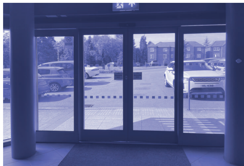
Fig.9 - Automatic sliding doors to reduce obstacles, with contrasting trim.
