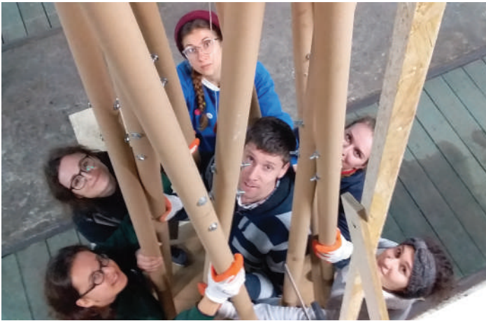
1. Assembly process of the tower.
