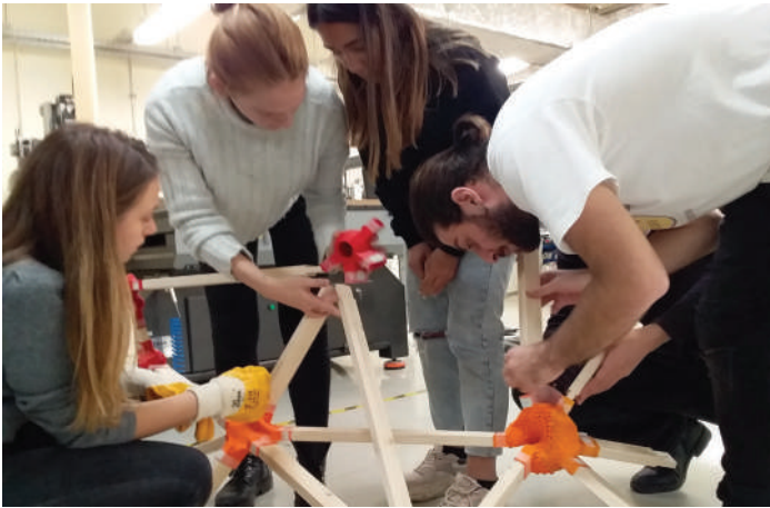
1. Assembly process of the beam section of The Gate.
