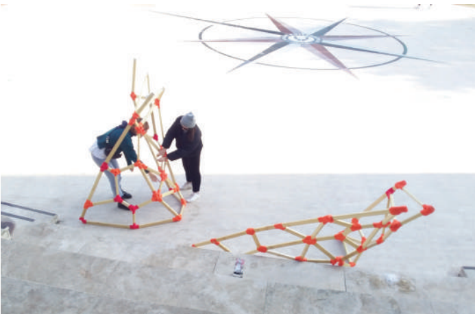
2. Last adjustments to the column sections before assembly.
