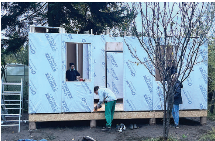
3. Assembly of the final prototype of the TECH 05.
