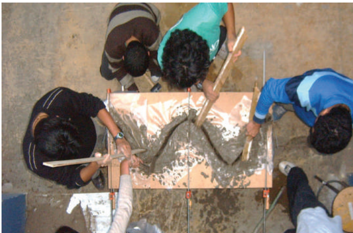
2. Fabrication of one of the models in reinforced concrete.
