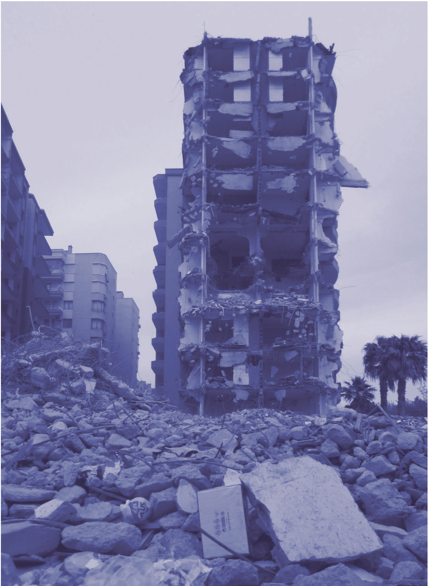
Demolition of buildings in Izmir..
