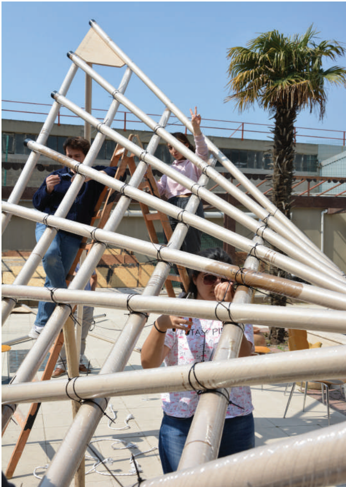
1. Assembly process of the structure.
