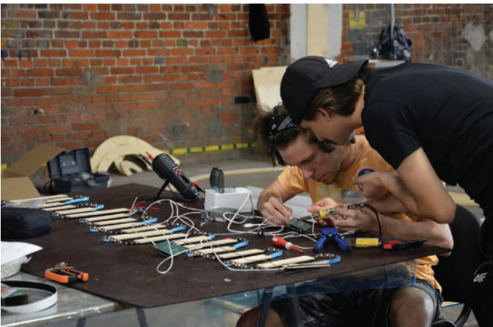
2. Electronic installation of the Reception Desk.
