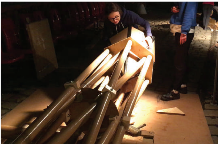
2. Fixing the last components of the tower before installation.
