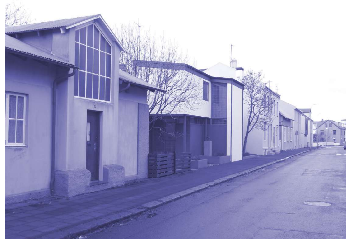
Fig.8 - The house is singular for its respect for the preexisting environment in grown street, receding from the street and creating a sheltering entrance from the wind and rain (© The Cultural Heritage Agency of Iceland)
