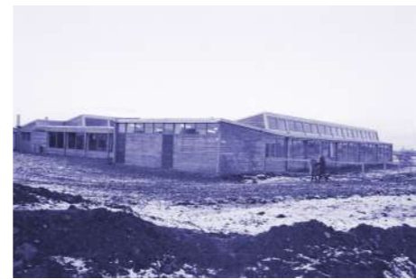
Fig.7 - Newly built Réttarholtsskóli, first phase. The construction started in May 1957 and teaching started in 8 classrooms the same autumn. Characteristic is the raw concrete and composition of windows, as well as how the light is brought into the building from above (© Reykjavík Photography Museum. Photographer: Pétur Thomsen 1910-1988).
