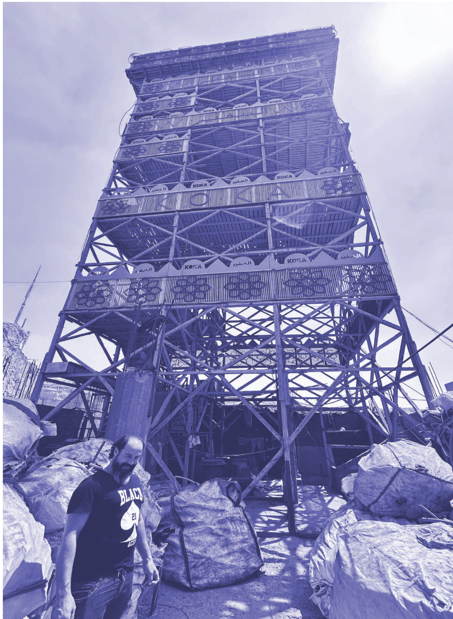
Fig.2 – Wasseem, the owner and the Koka Tower. Copyright to the author.
