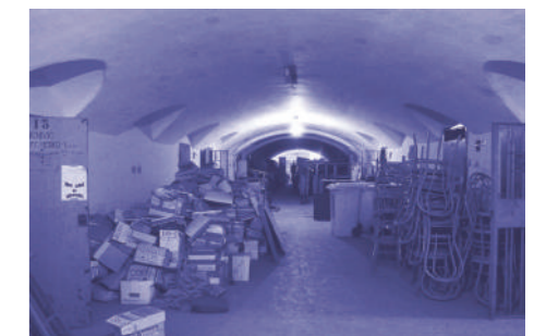
Fig.7 - ReverseLab , the first ray basement before the renovation work.
