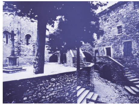
Fig.1 - "The contact space" Saint Martin of Londres. Romanesque church and surrounding wall of the former priory. CHOAY, F. Spazi Urbani nel Tempo. Skira, 2003, p 23.
