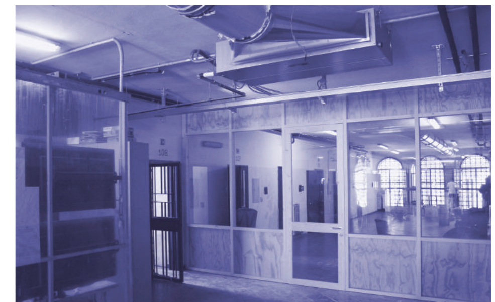
Fig.6 - The ongoing works within the CAR section.
