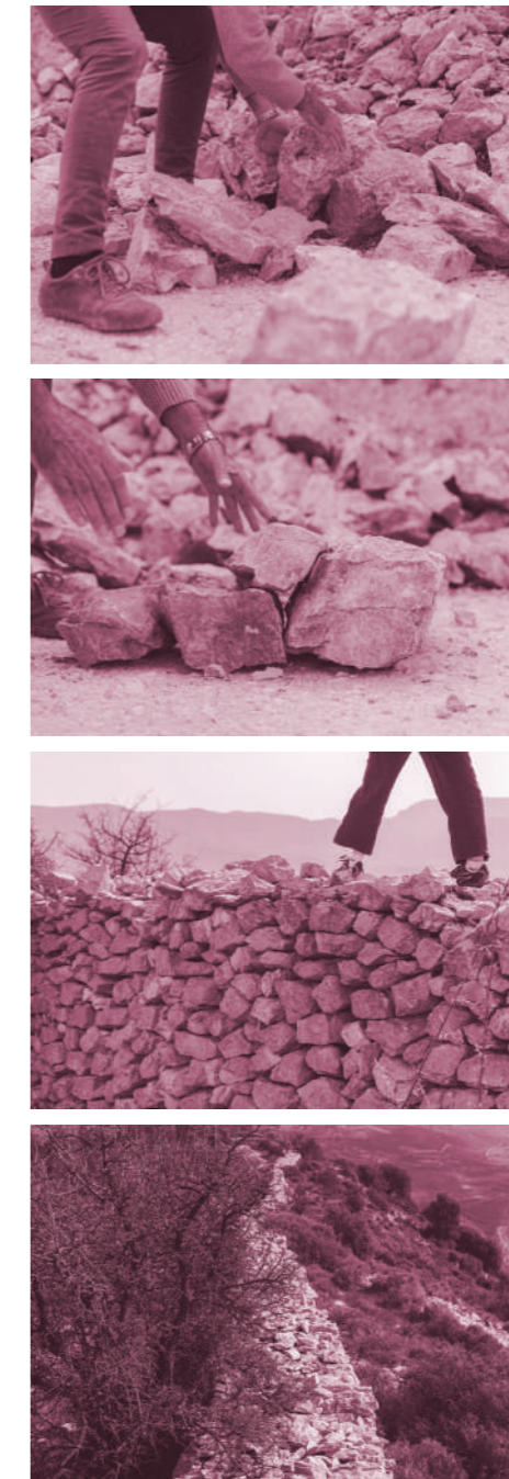
Fig.2a,b,c and d - The process of drystone assembling scaled in 'The Measure of the Land'. 2
