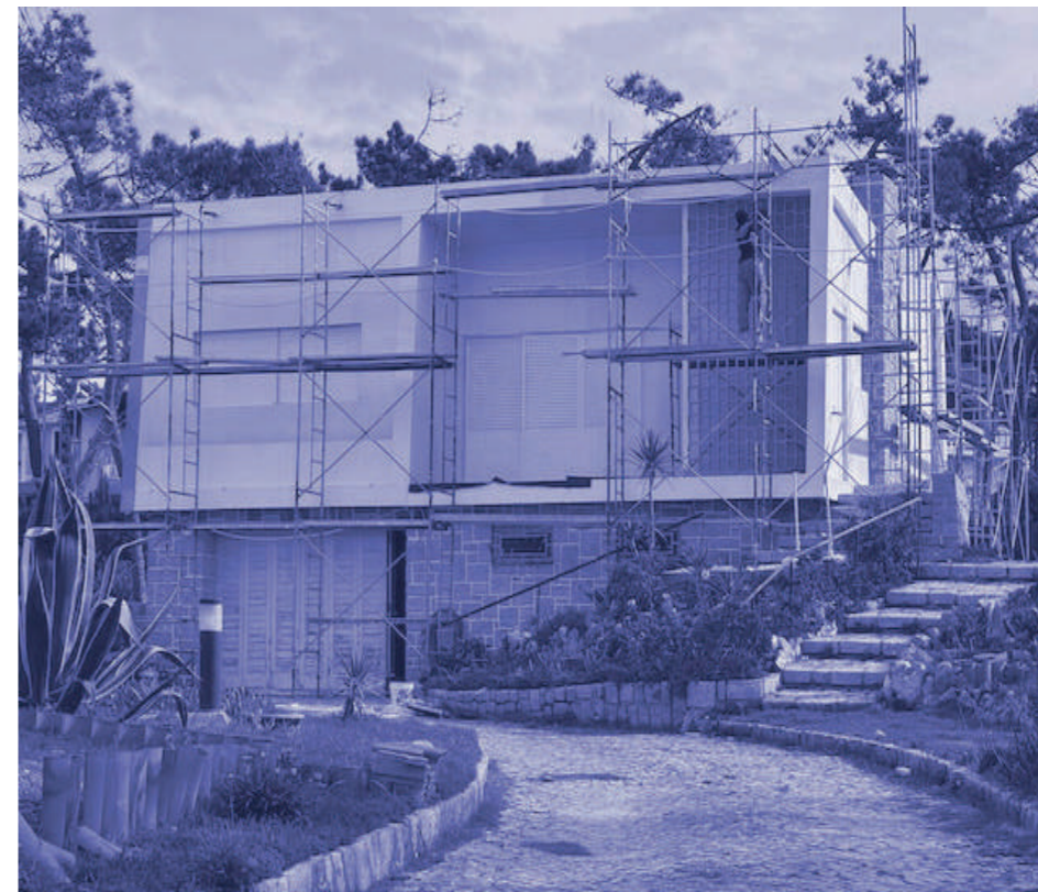
Fig.5 - The same house during intervention, November 2025. Uniform white replaces the original chromatic differentiation. New window profiles designed for continental thermal performance occupy openings calibrated for Atlantic light. The building permit's promise — 'simple and without artifice, valorised by different materials and colours' — is being overwritten in real time. Source: author, 2025.
