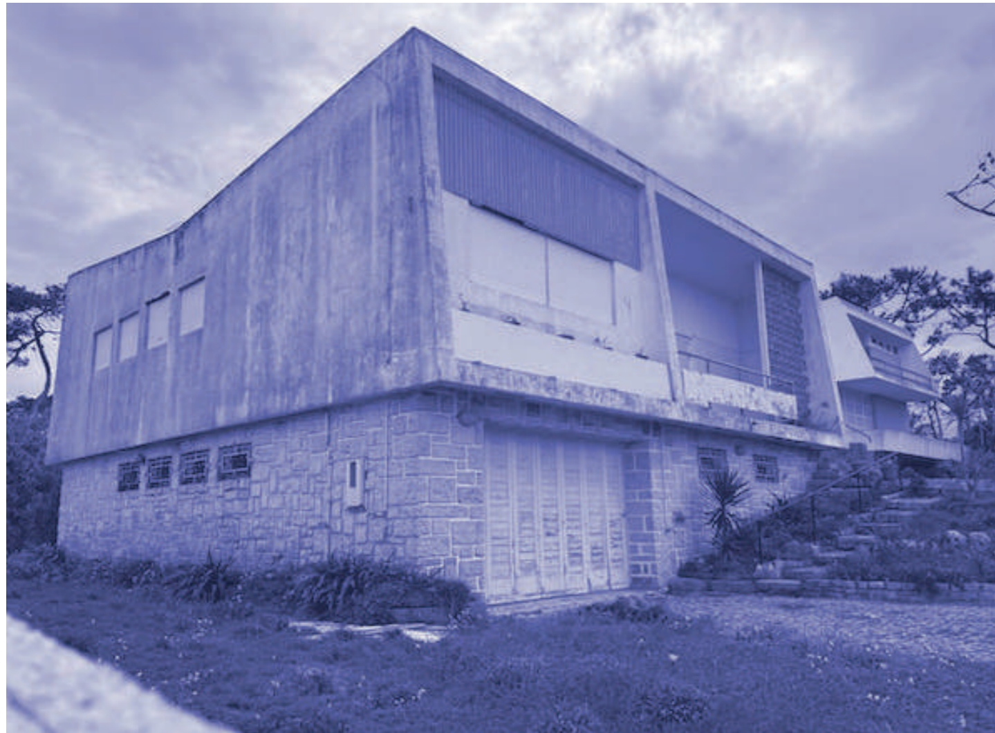
Fig.3 - The same house, 2024. Material weathering has advanced — concrete staining, paint erosion — but the architectural script persists: volumetric articulation, proportional openings, the dialogue between stone base and rendered upper volume. The house ages; it does not yet dissolve. Source: author, 2024.
