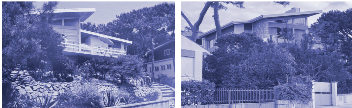
Fig.6 - Summer house on the slope (Sections 1 and 6), composite. Left: original state — tubular steel balustrade, wire mesh, timber soffit, terraced garden. Right: current state — frameless glass, stainless steel fixings, metal gate. The structure endures; the script has been overwritten. Sources: private archive (left); author, 2024 (right).
