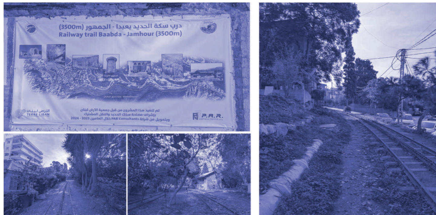
Fig.7 - Left to right: The plan of the Railway Trail in Baabda opened by Terre Liban Association. Stretches of the opened trail with the visible train tracks, and the old Baabda train station in the 2nd picture in the bottom row. Photos by the author, January 2026.
