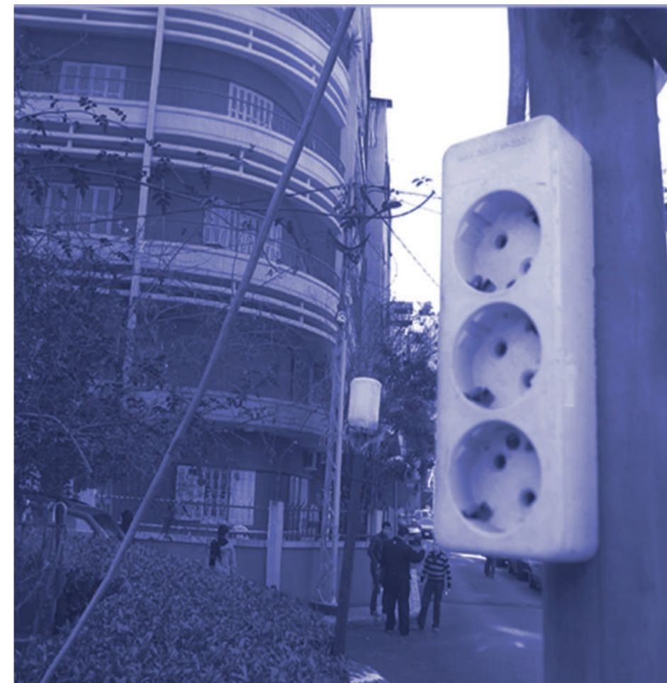
Fig.9 - Lighting pole and electricity socket (2012).
