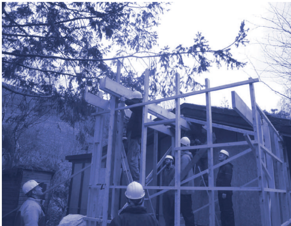
Fig. 3. Contemporary example of the Segal construction method in use. Photography by Cay Green
