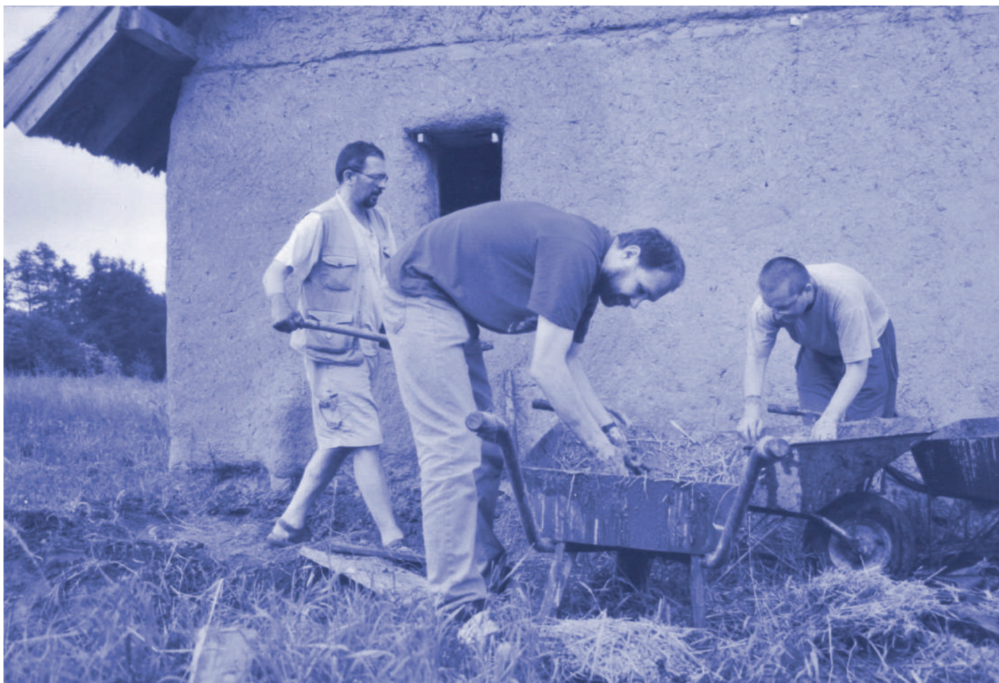
Figure 9. Direct contact with material and building processes is a characteristic of many low-tech constructions. In the picture: the author (in the forefront) mixing cob for Kadłubówka first Polish straw-house design by Paulina Wojciechowska
