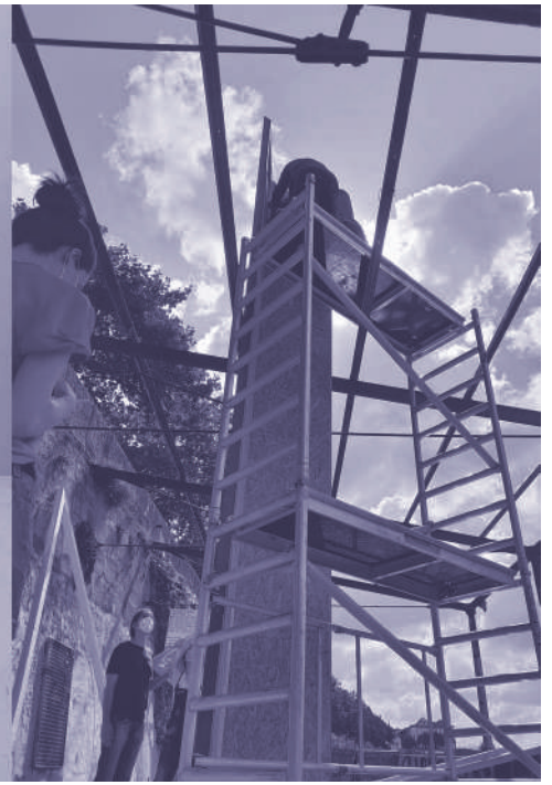
Fig. 7 - Petite Folie #6 work in progress.
