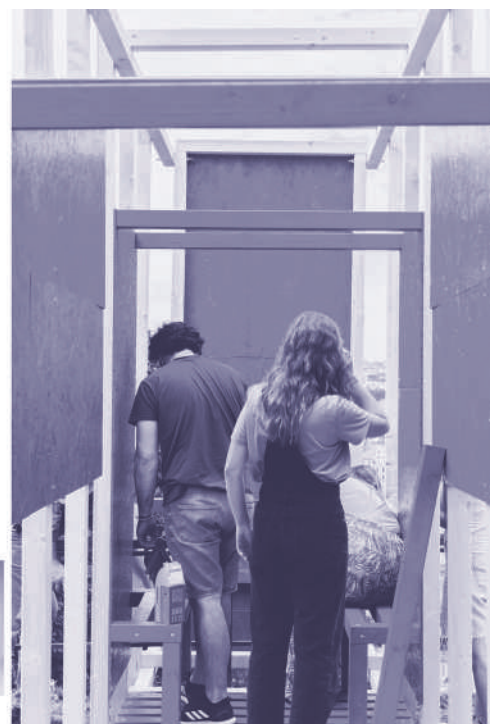
Fig. 6 - Petite Folie #4 work in progress.
