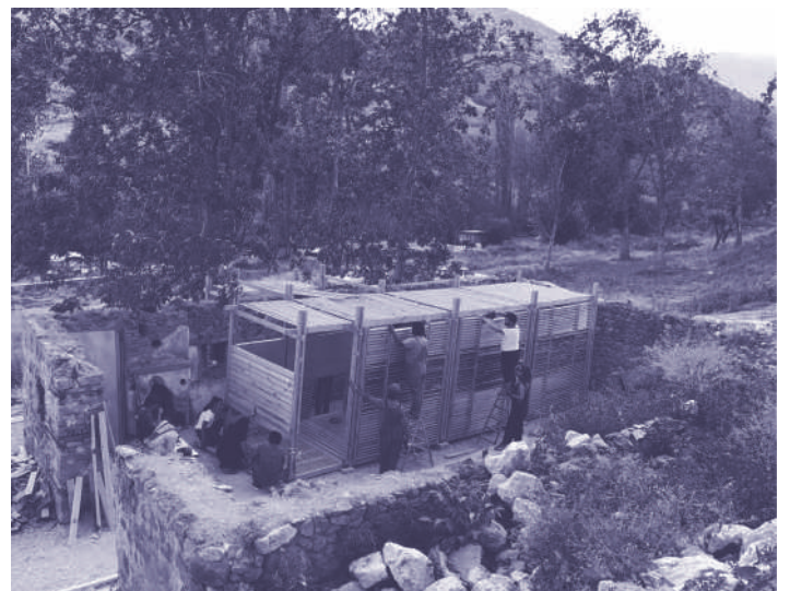
Fig. 3 - Construction of the folie, Merzifon, 2017
